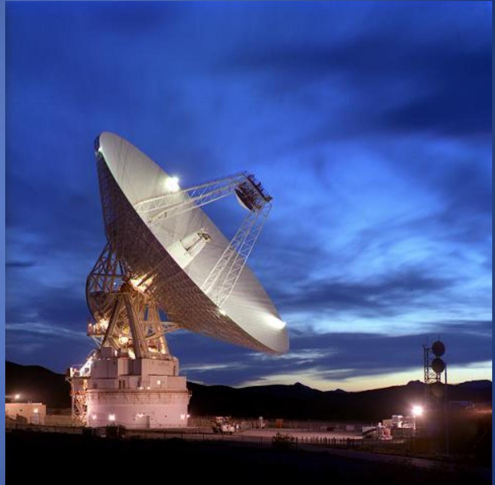
A 70-meter dish antenna. Part of NASA's Jet Propulsion Laboratory (JPL) communication system.
