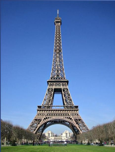
In 1913, the Eiffel Tower was used as an antenna. Back when communication was at very low frequencies, the antennas had to be very large to get any sort of radiation. The Eiffel Tower fit this bill well, and was used to communicate with the United States Naval Observatory in Arlington, Virginia.
